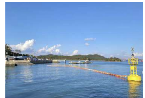
Installation of an anti-pollution screen to protect otter food sources
