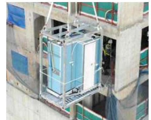
Installation of prefabrication bathroom unit (PBU)
